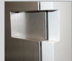
Notch-type access port in door
